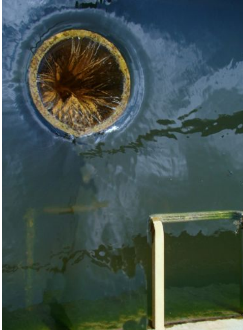
Figure 3 – Rosethorne effluent structure, mid June 2010
